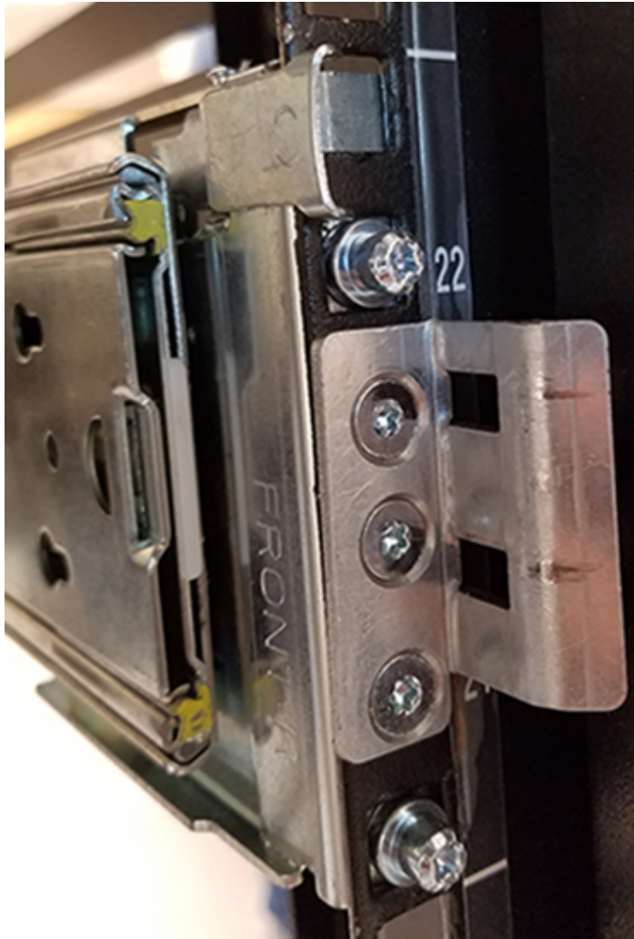
Figure 140: Rack Latch Bracket Installed
